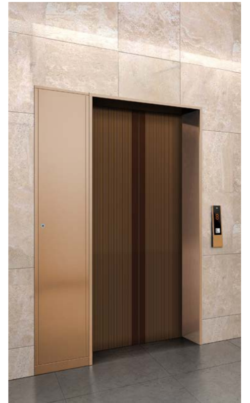
Entrance with control panel
