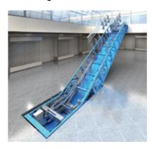
Installation of central modules, track system and step band, and alignment through laser to ensure a perfect fit for a smooth ride and low noise levels.
