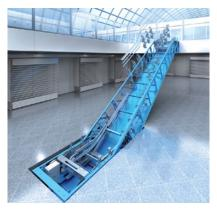
Installation step 3 – Middle segment Install central modules, track system and step band. Align to ensure a perfect fit.
