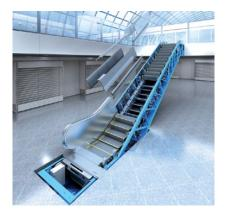
Installation step 4 – Aesthetic upgrade Install visible components such as balustrade, decking, cladding, if applicable, and floor plates to make escalator look like new.
