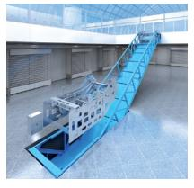
Installation step 2 – Installation Install components, including electrical cabinet and distribution boxes. Align new upper and lower modules using adjusting tools.
