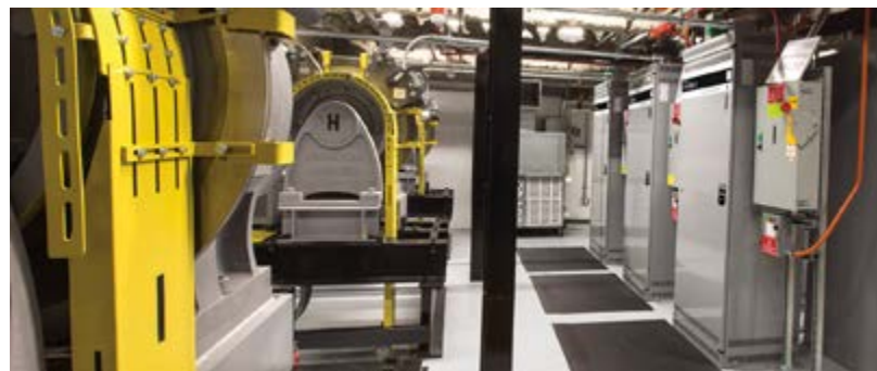
Pictured: Top, a modernized lobby with upgraded Destination Control and fixtures. Bottom left, a modernized door with UDO upgrade. Middle, an upgraded machine room with new machines and controllers. Bottom right, modernized roller guides.
