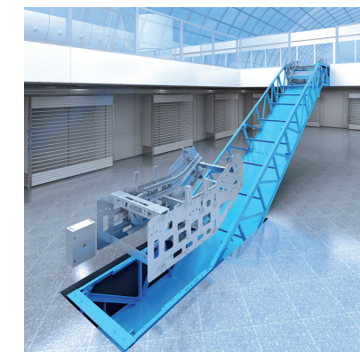
Installation step 2 – Installation Install components, including electrical cabinet and distribution boxes. Align new upper and lower modules using adjusting tools.
