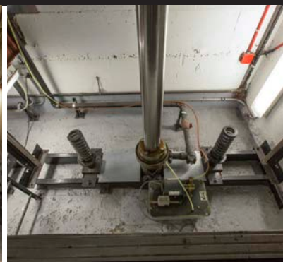
Hydraulic elevator modernization
