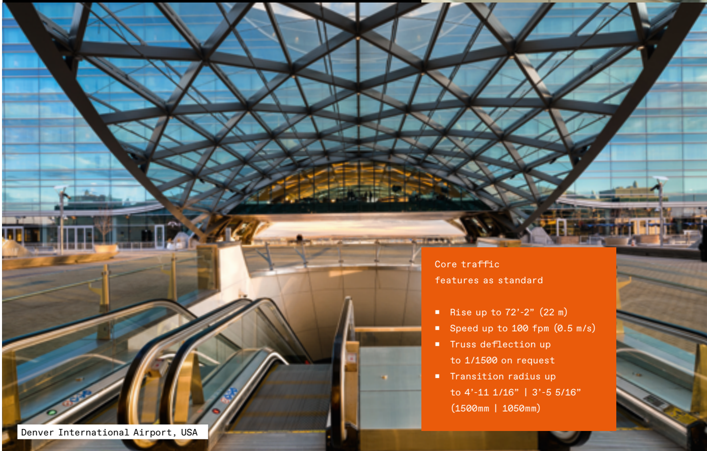
Denver International Airport, USA
